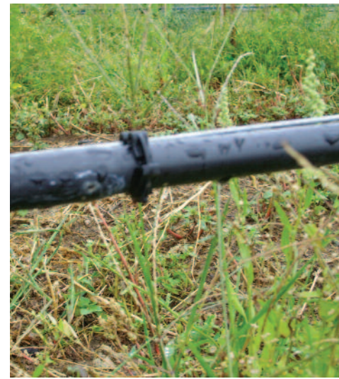
OVER GROUND DRIP IRRIGATION
